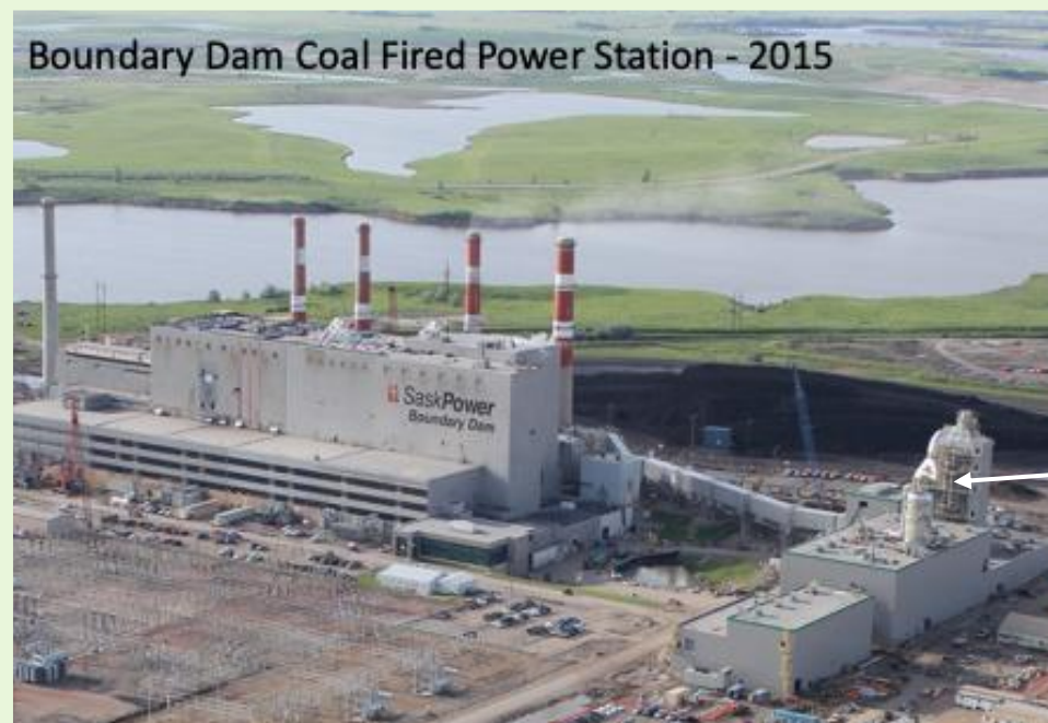
Packed CO 2 absorber column
